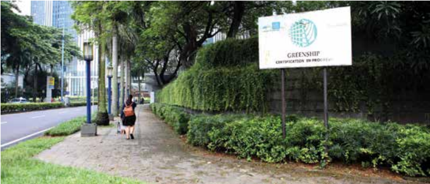
Certified building Gold Standard Certificate for Green Building.
