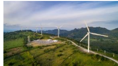
UPC Sidrap Bayu Energi, First Wind Power Plant in Indonesia. (2020)
