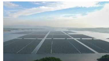
Cirata Floating Power Plant, Largest Floating PP in Indonesia (2021)
